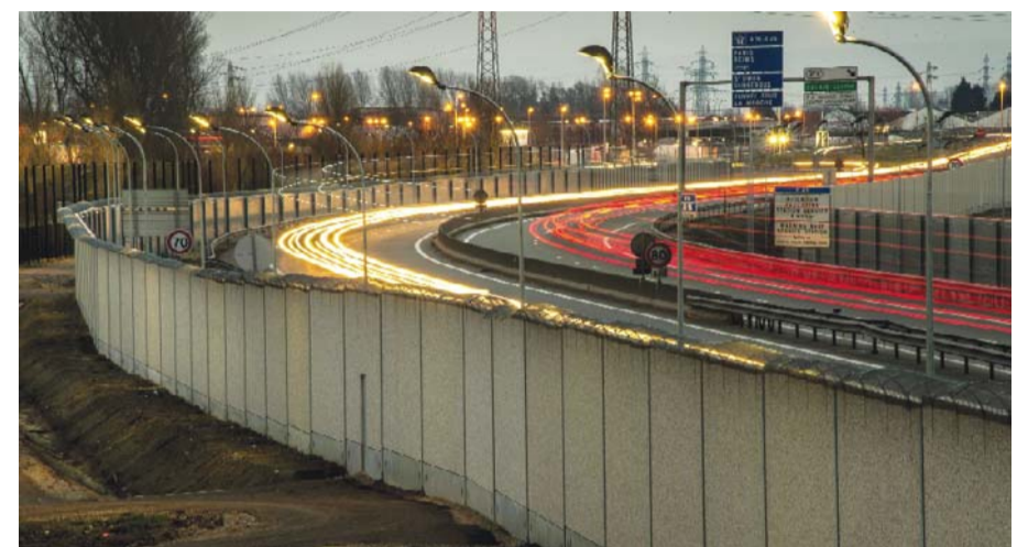
This photo taken on Feb 2, 2017 shows a four-metre-high wall running along a kilometre-long stretch of the main road leading to Calais port, aimed at stopping migrants who attempt to reach its shores.
