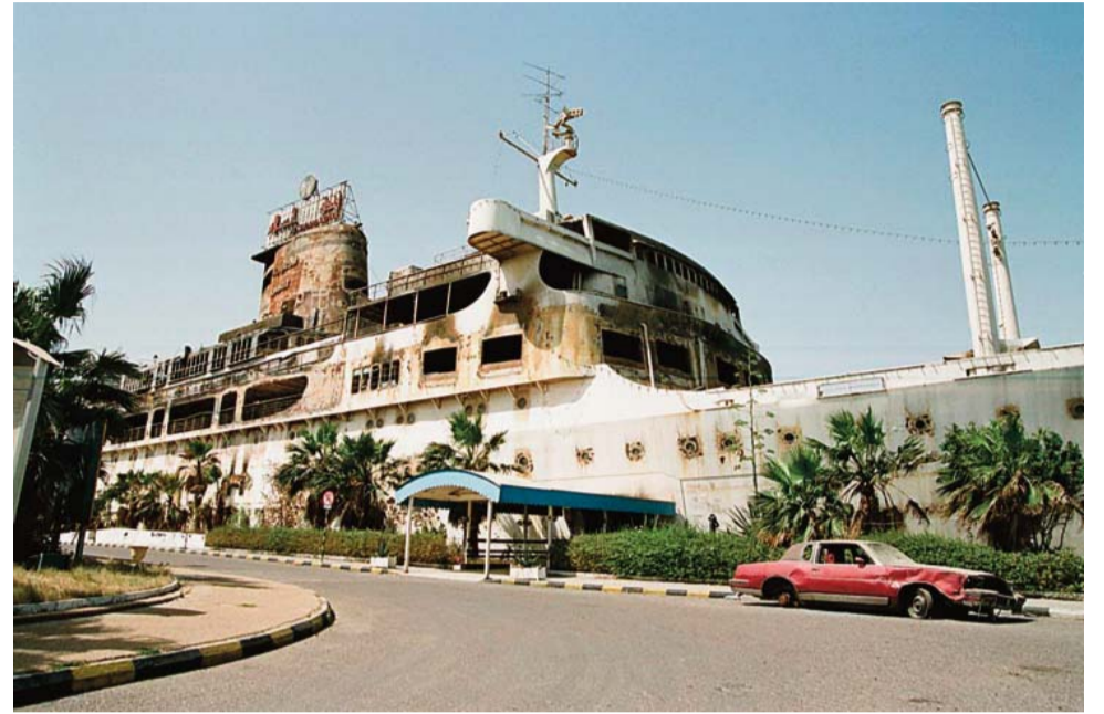
Iraqi forces completely destroyed the Ramada Al-Salaam Hotel; a passenger/cargo ship-turned-five-star hotel in Kuwait City.
