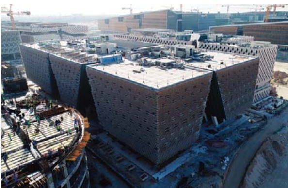
Ongoing construction works at the Sabah Al-Salem University City.
