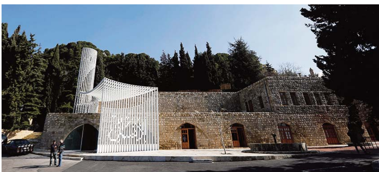
The exterior of the Amir Shakib Arslan mosque designed by Lebanese architect Makram El-Kadi at the entrance of the Druze heartland village of Mukhtara in Lebanon's Chouf mountains. — AFP photos
