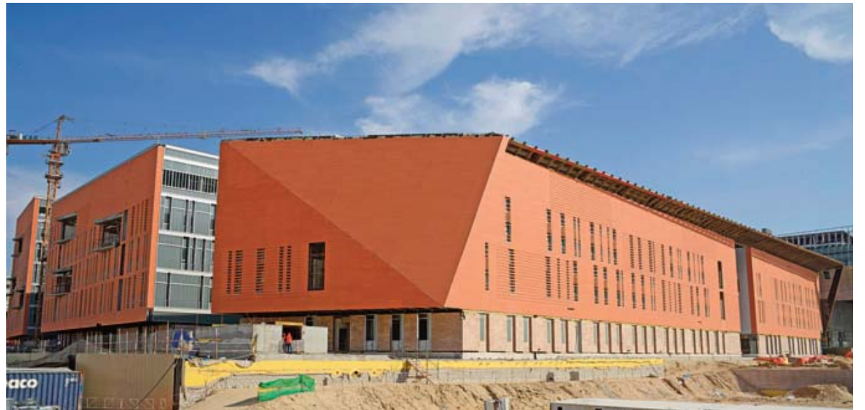
A building under construction at the Sabah Al-Salem University City.
