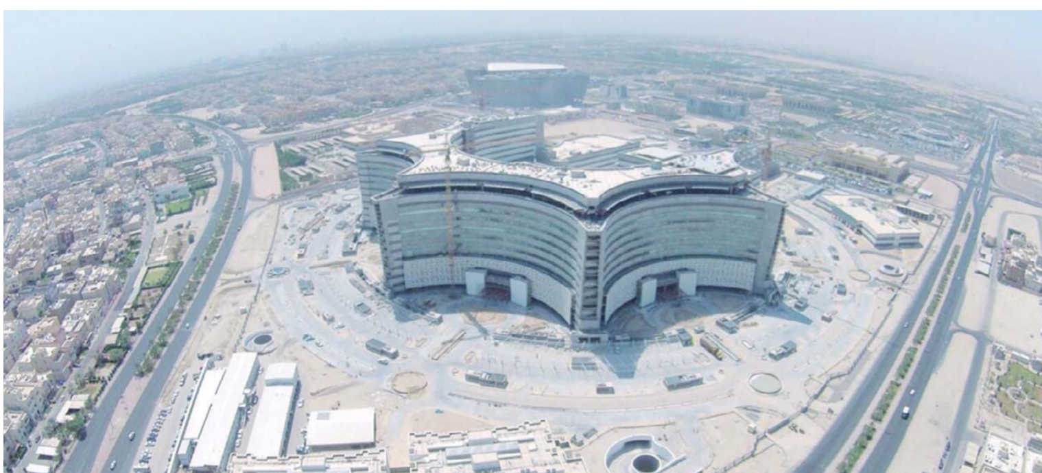
KUWAIT: This file photo shows the Jaber Hospital under construction. The hospital, one of the largest in the Middle East, will serve Kuwaiti citizens exclusively when it opens later this year. MP Ahmad Al-Fadhil believes this nationality-based segregation is wrong.
