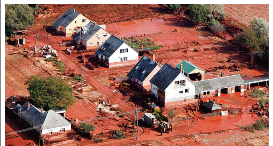
KOLONTAR, Hungary: An aerial view of the village of Kolontar, nearby the Torna stream, some 160 kilometers southwest of the Hungarian capital Budapest, after a wave of toxic red mud of the Ajkai Timfoldgyar plant swept through the village.
