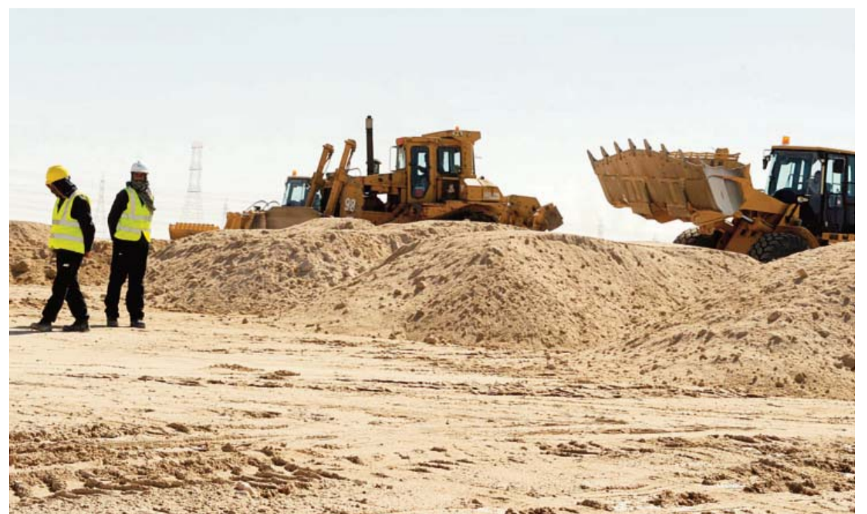
Ongoing construction works at the South Mutla City project.
