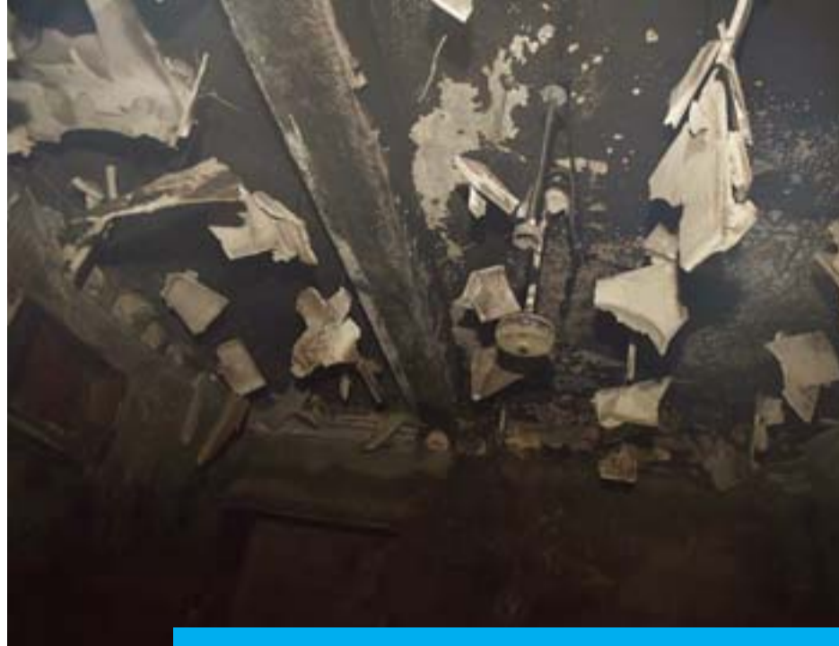
KUWAIT: The gutted house in Sabah Al-Salem.
