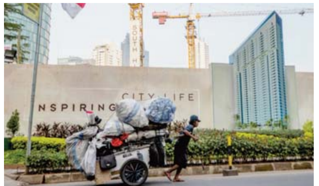
JAKARTA: A worker pulls his fully-loaded cart past an apartment complex under construction in Jakarta yesterday. — AFP
