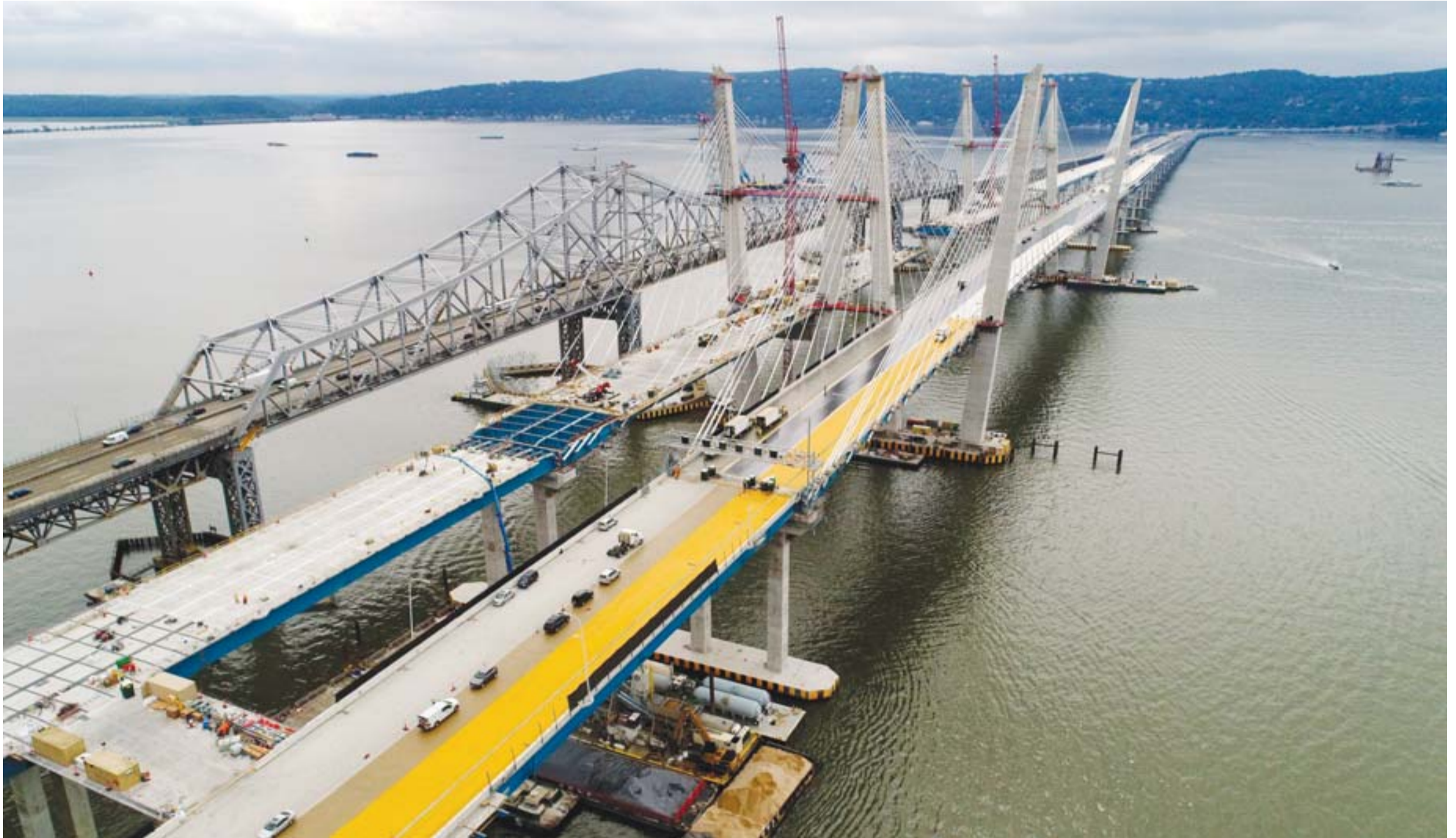
In this July 25, 2017 file photo, construction continues on the spans of the new Governor Mario M. Cuomo Bridge, right, as vehicles make their way on the Tappan Zee Bridge over the Hudson River, near Tarrytown, N.Y. President Donald Trump's road to getting legislation through Congress this year to restore the nation's crumbling infrastructure appears increasingly precarious. — AP
