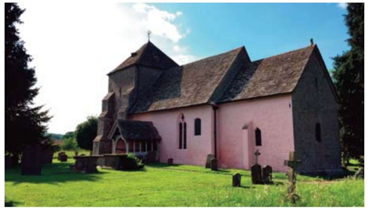
Photo shows St Mary's Church at Kempey, in Gloucestershire, western England.
