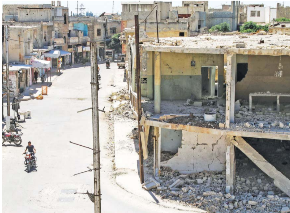
TALBISEH: A man rides a motorcycle down a street past a damaged building in the central Syrian rebel-held town of Talbiseh, north of Homs. — AFP
