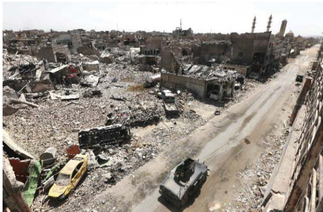
MOSUL: A picture shows damaged buildings in the old city in western Mosul.—AFP
