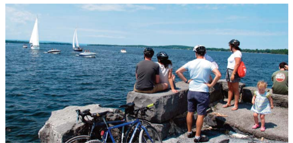
Bicyclists watch as boats prepare to pass through a cut in an abandoned railroad causeway from the Vermont mainland to the Lake Champlain islands.
