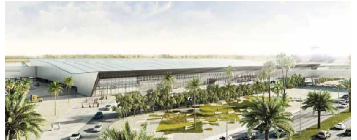
The support terminal.
