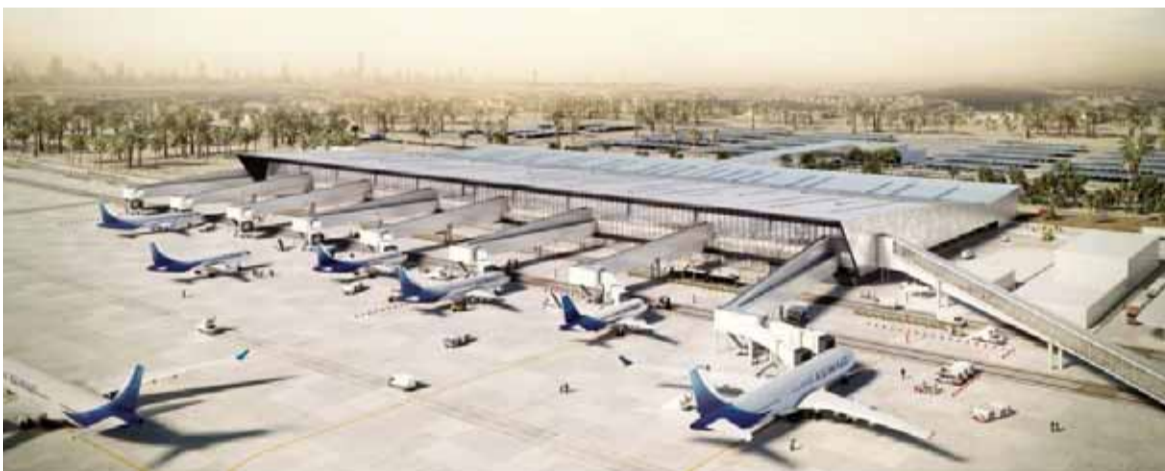
An artist's rendition of the Support Terminal, to be implemented as part of Kuwait International Airport's development project.
