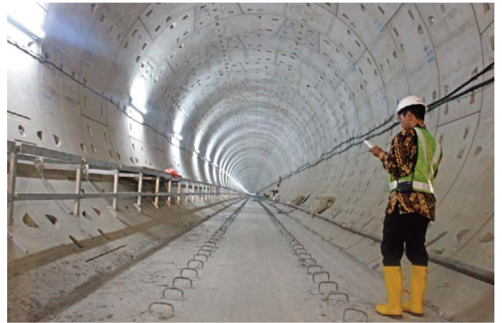
Metro project in process in Jakarta
