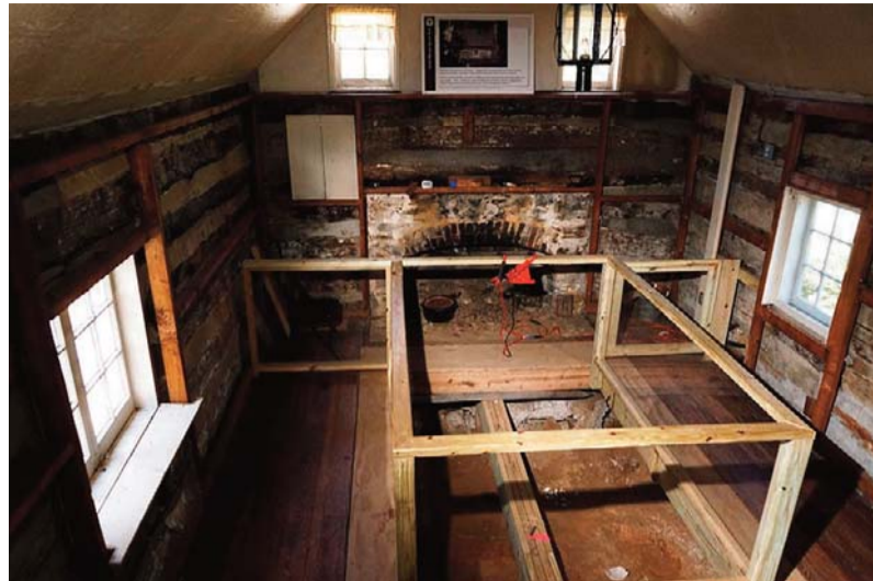
The interior of a log cabin structure which was originally used as a kitchen, next to the plantation house at Josiah Henson Park in Bethesda, Maryland.
