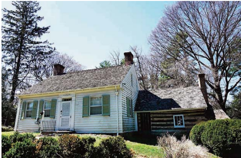
Photo shows the log cabin structure which was originally used as a kitchen, next to the plantation house at Josiah Henson Park in Bethesda, Maryland.
