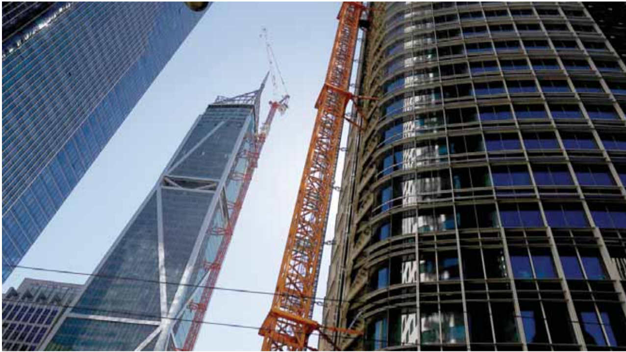
CALIFORNIA: Construction cranes are seen on two buildings that are under in San Francisco, California. —AFP
