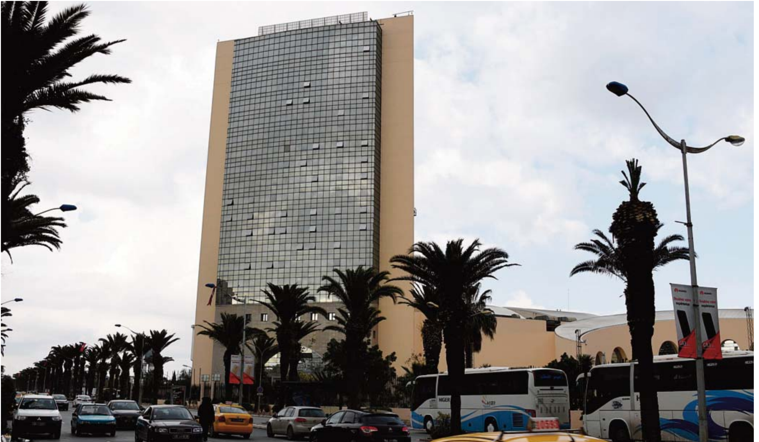
TUNIS: Photo shows the abandoned headquarters of ousted Tunisian president Zine El Abidine Ben Ali's Constitutional Democratic Rally party (RDC) in central Tunis. The make-over of the former RDC headquarters is nearly complete and it will soon be operational - hosting three ministries. —AFP
