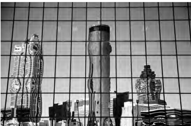
ATLANTA: The Westin hotel, center, is reflected along with other downtown buildings in the windows of an office tower on Wednesday.—AP
