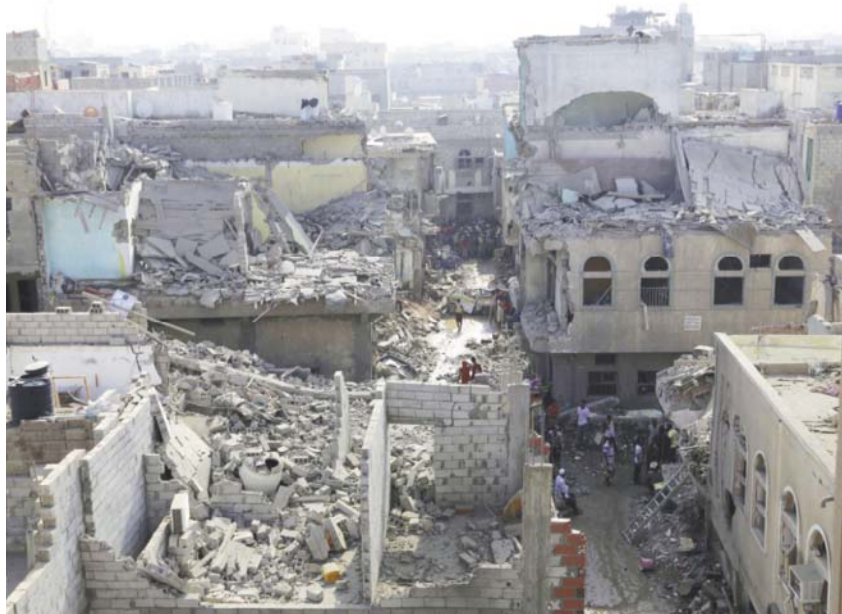
HODEIDAH, YEMEN: A general view shows buildings destroyed during Saudi-led air strikes yesterday. —AFP
