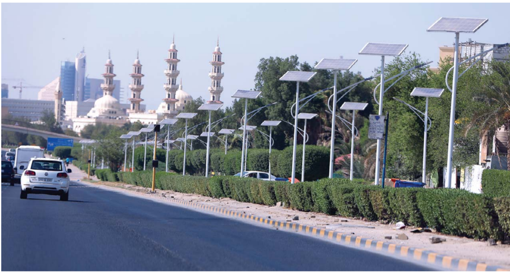
KUWAIT: Photo shows solar panels lining the walking track in the Kuwait neighborhood of Khaldiya. Solar panels to generate electricity have been installed in several areas around Kuwait in recent months in a bid to reduce reliance of fossil fuels and improve Kuwait's energy profile. — Photo by Yasser Al Zayyat
