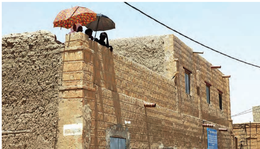
Residents watch from a rooftop as the doors of a revered 15th-century mosque.
