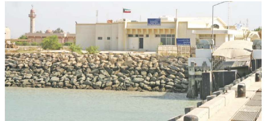
The Failaka port currently under renovation.
