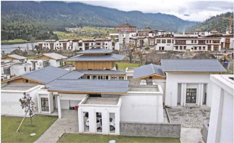
A construction site behind chalets of the Artel hotel in Lulang, near Nyingchi in China's Tibet Autonomous Region. — AFP photos
