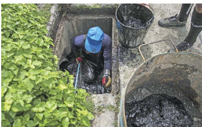
BANGKOK: A volunteering prisoner inside a drain channel during an operation to dredge it from sewage and plastic waste.
