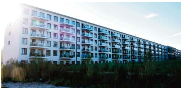
A construction site of luxury apartments as part of transformation of the heritage-protected Prora Complex.
