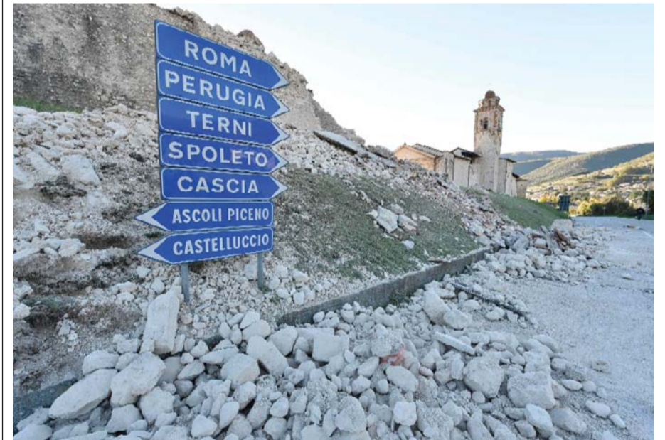
NORCIA, Italy: Picture shows damage near the center of this town following a 6.6 magnitude earthquake yesterday. — AFP
