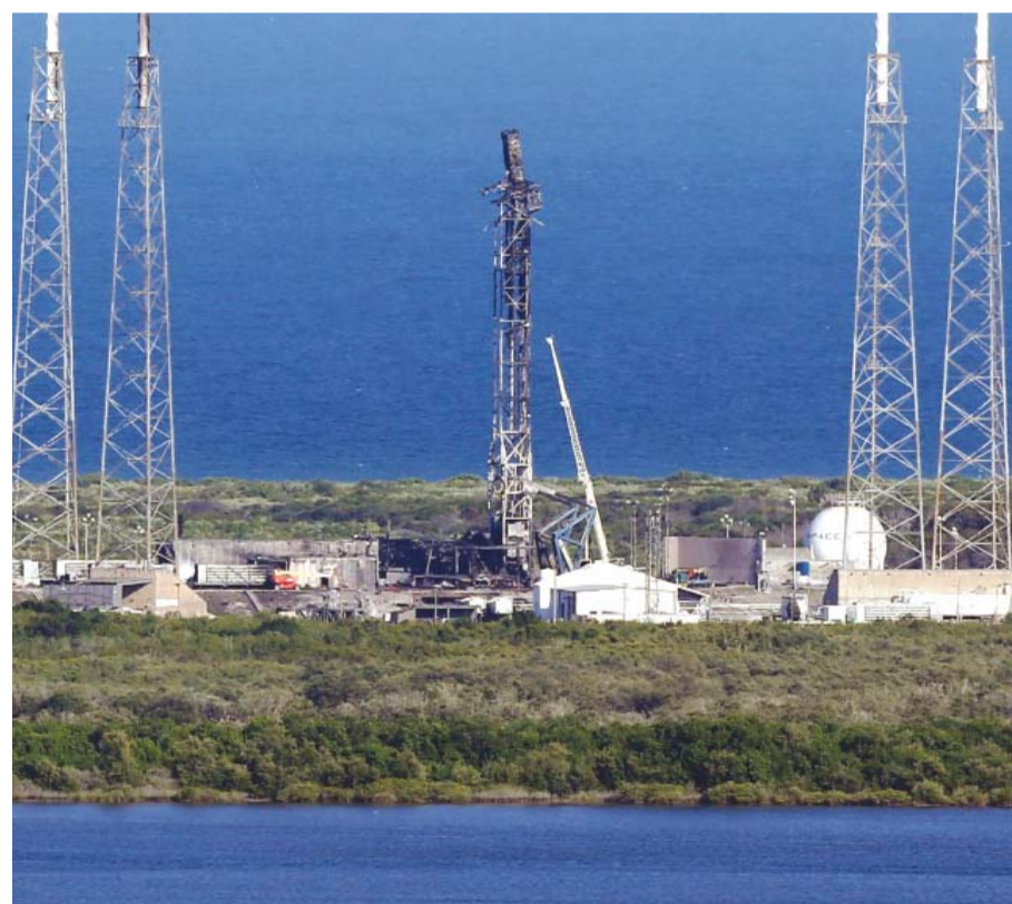
This Thursday, Sept. 8, 2016 file photo shows the damaged SpaceX launch complex 41 at Cape Canaveral Air Force Station in Florida. — AP
