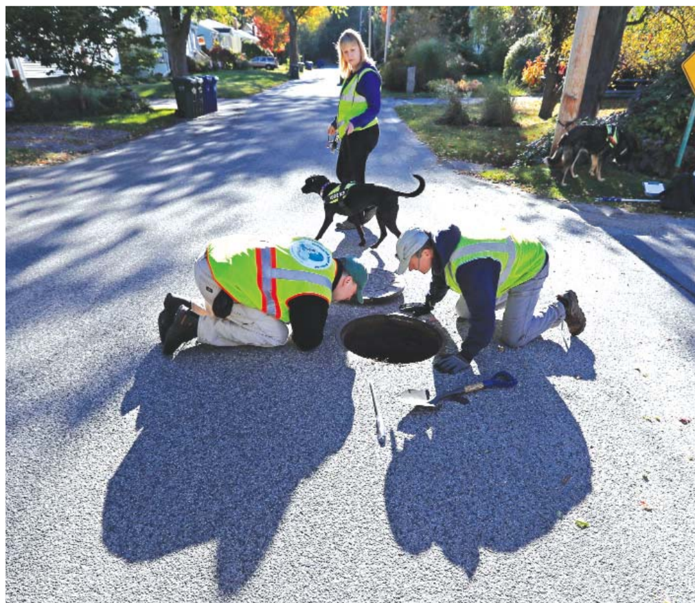
SOUTH PORTLAND: In this Tuesday, Oct 11, 2016, photo, Scott Reynolds of Environmental Canine Systems, left, and Fred Dillon, the storm-water program coordinator for the city of South Portland, Maine, inspect a storm water drain pipe. — AP
