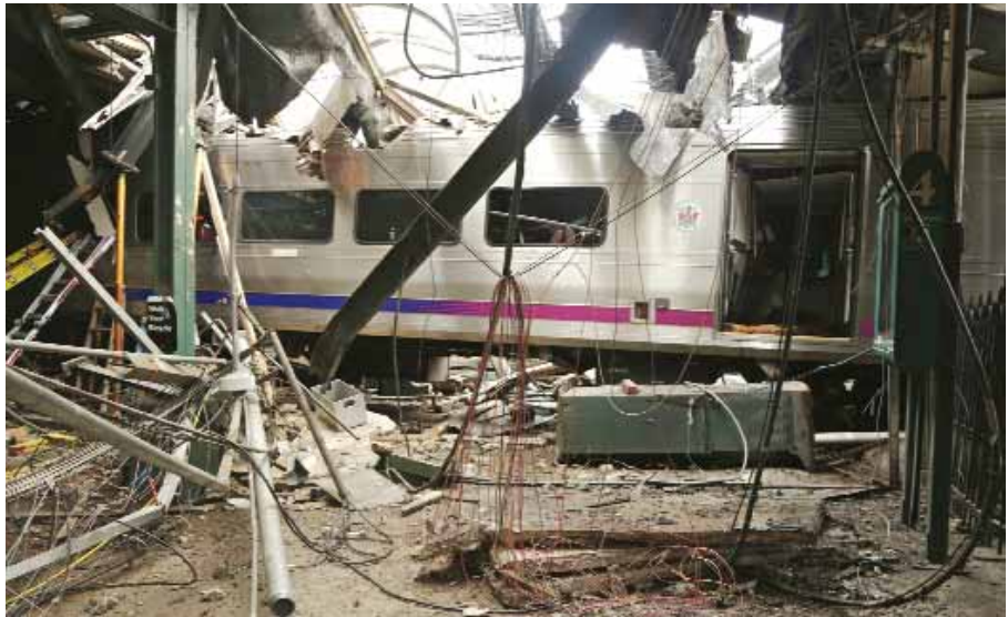
HOBOKEN, NEW JERSEY: This Oct. 1, 2016, file photo provided by the National Transportation Safety Board shows damage done to the Hoboken Terminal.—AP
