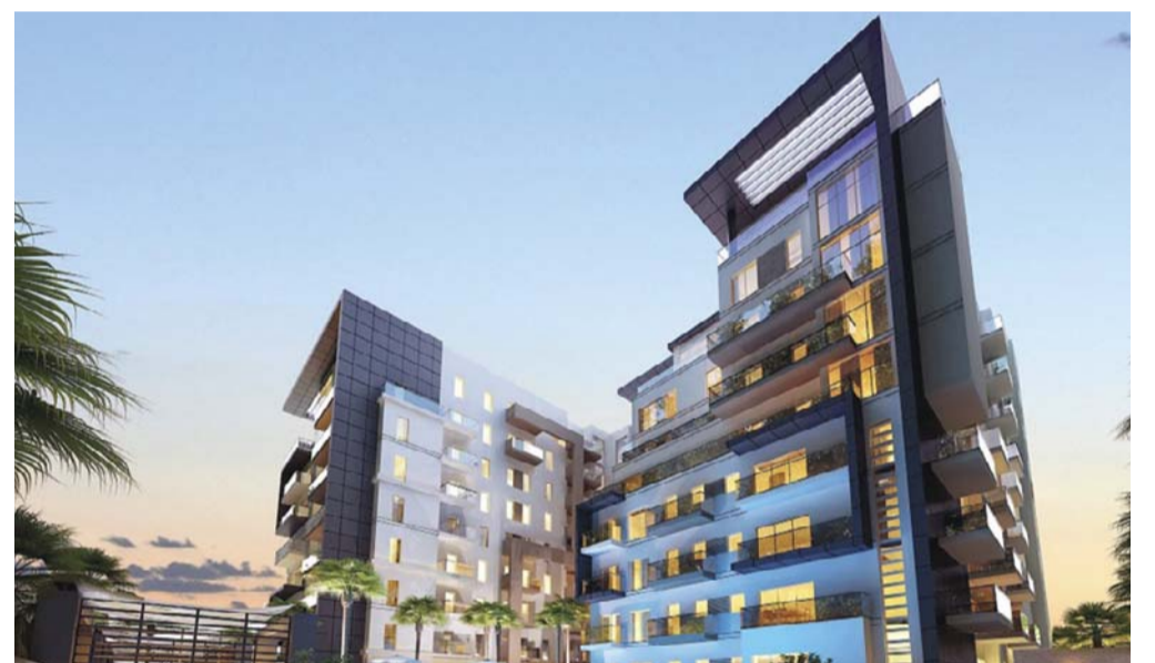
DUBAI: First project completed in Dubai South — DAMAC Maison de Ville Tenora.
