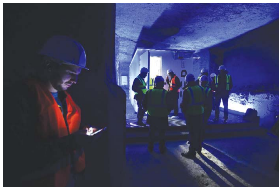
SAUMUR, France: A man looks at his cellphone as people visit a room of cabling servers in an underground datacenter yesterday near Saumur, western France. The underground datacenter is built in a former quarry in order to maintain a low temperature for the servers and consume less electricity. —AFP
