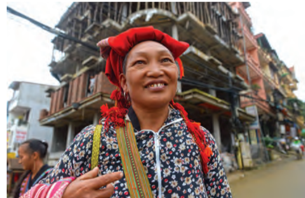
A Dao ethnic woman selling tourist souvenirs in front of a new hotel under construction in the northern Sapa tourist town.
