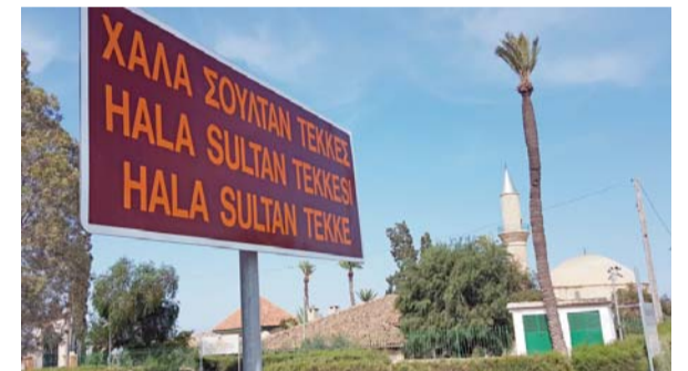
Hala Sultan Tekke Mosque.
