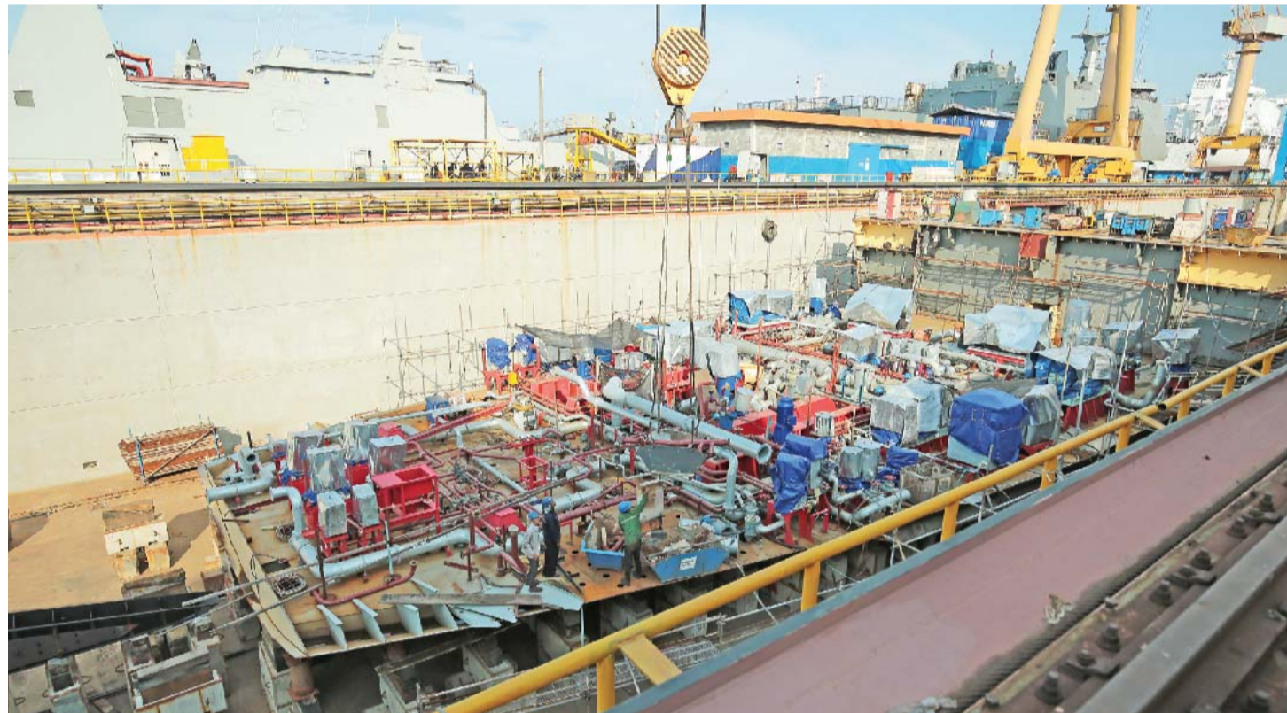
The Surabaya shipbuilding factory.
