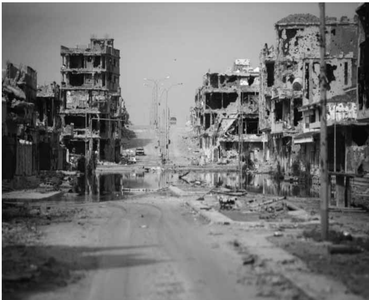
SIRTE, LIBYA: A general view of buildings ravaged by fighting.—AP
