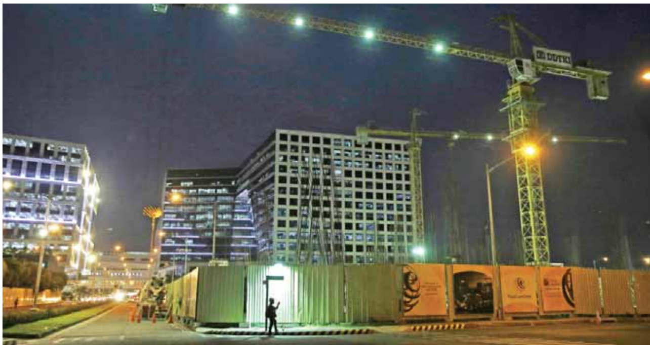
MANILA: A Filipino worker checks his phone as he waits outside a construction site at a commercial area in suburban Pasay, south of Manila, Philippines, yesterday. The Philippine economy grew faster than expected at 6.9 percent in the first quarter from the same period a year ago, its highest quarterly growth in almost three years, officials said yesterday as the government prepares to hand over leadership to the incoming administration. — AP
