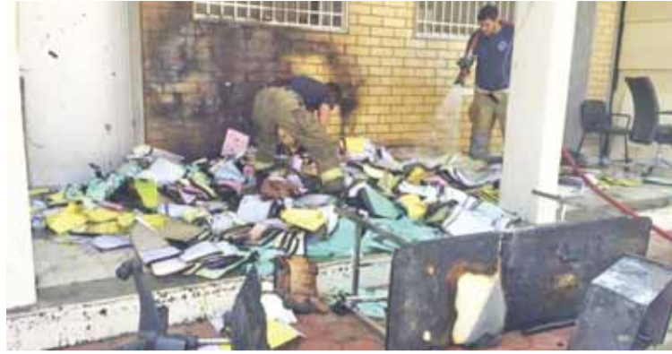
KUWAIT: Firefighters inspect damage after tackling a blaze at Qairawan Health Center yesterday.
