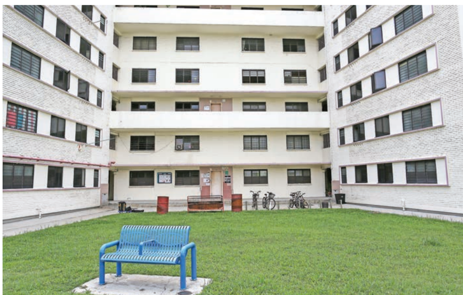
SINGAPORE: The residential block where an apartment registered to a Singaporean company "Black Tidings" is seen. — AP
