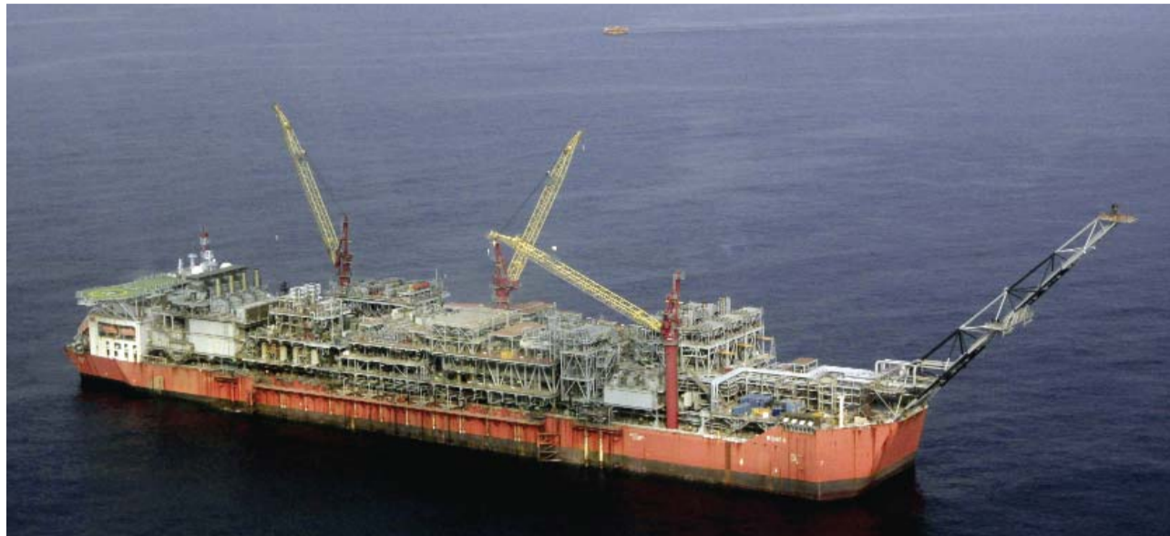
Shell Bonga offshore oil Floating Production Storage and Offloading vessel off the coast of the Niger Delta in Nigeria. Shell closed the terminal exporting Nigeria's benchmark Bonny Light crude oil on Wednesday and was evacuating workers from a threatened oil field as renewed militant attacks cut production in Africa's biggest petroleum producer, the company and a union leader said. — AP
