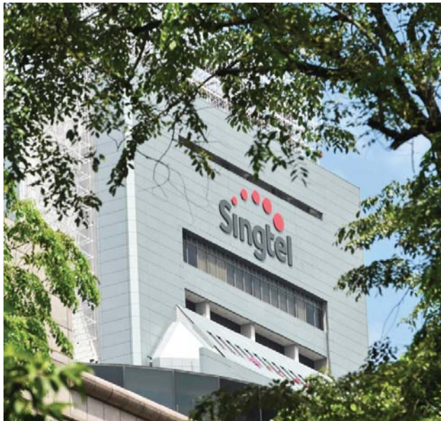
SINGAPORE: Singtel logo is seen on its headquarter building in Singapore yesterday. — AFP
