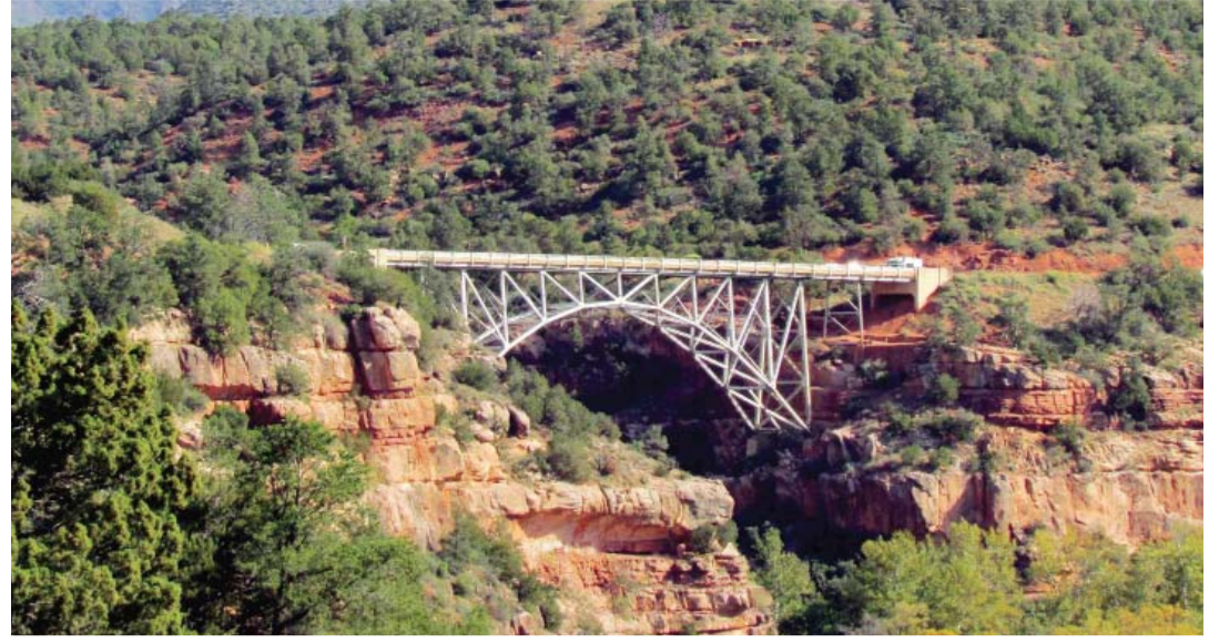
ARIZONA: This undated photo shows Midgely Bridge in Sedona. — AP
