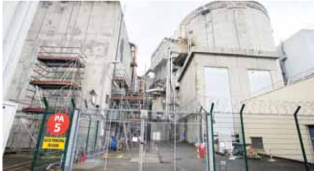
FESSENHEIM, France: This file photo taken on April 09, 2013 shows a reactor of the Fessenheim nuclear power plant. — AFP
