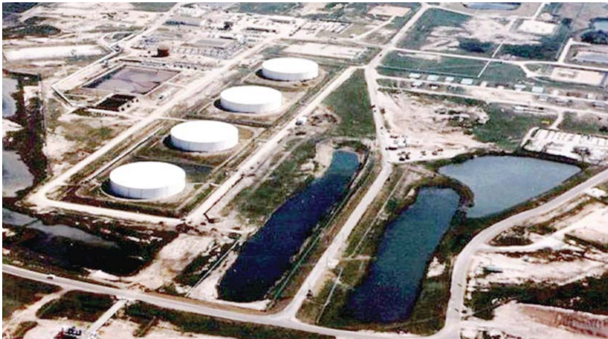
The US Strategic Petroleum Reserve (SPR) Bryan Mound storage facility located in Brazoria County.
