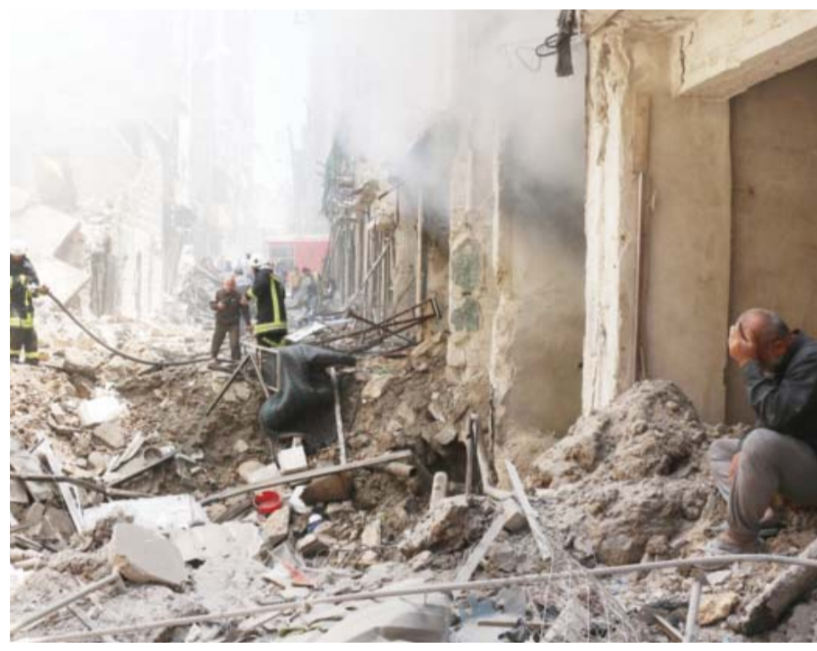
ALEPPO: A man sits on the rubble of a destroyed building following reported air strikes by government forces in the rebel-held Shaar neighborhood of the northern city Aleppo yesterday. — AFP
