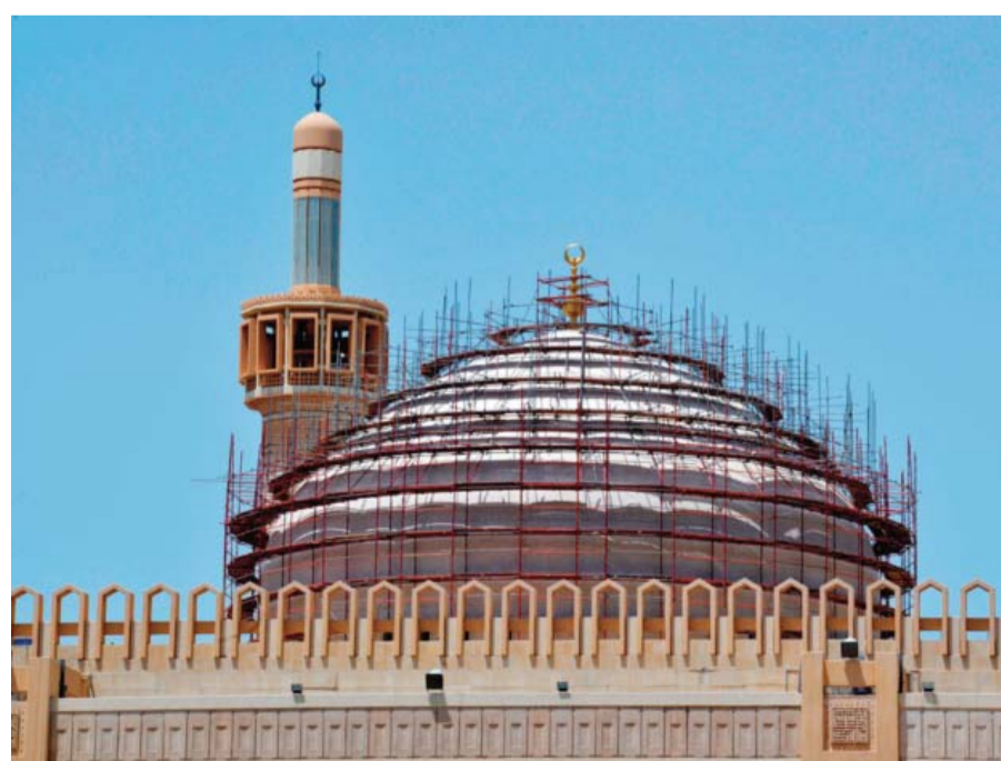
Renovation works at the Grand Mosque's dome.
