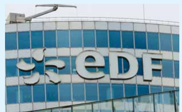
PARIS: The EDF tower of French state-owned power giant Electricite de France (EDF), is seen in the La Defense business district. —AP
