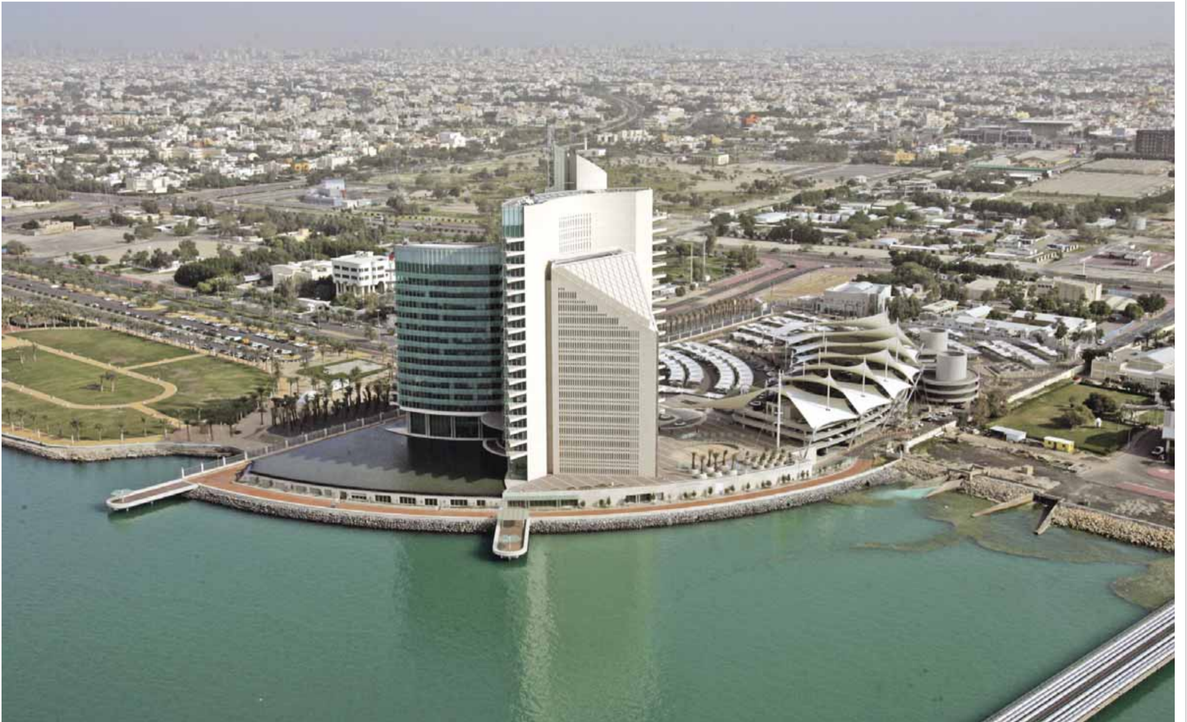
KUWAIT: The head office building of Kuwait Petroleum Corporation (KPC) in Shuwaikh. — KUNA photo
