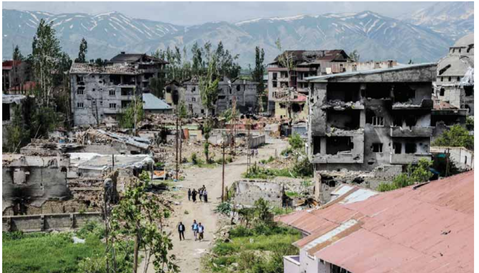
HAKKARI: This file photo taken on May 30, 2016 shows a general view of damaged buildings following heavy fighting between government troops and Kurdish fighters after the curfew on May 30, 2016 in the majority Kurdish city town of Yuksekova. — AFP
