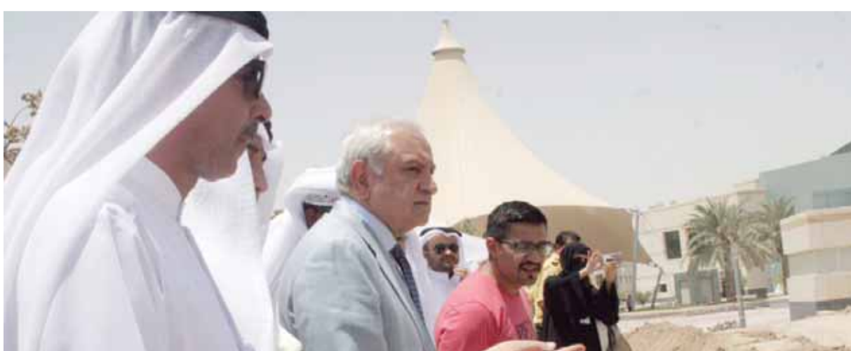
KUWAIT: Minister of Education and Minister of Higher Education Dr Bader Al-Essa yesterday inspected the scene where a roof recently collapsed at a multistorey car park, affiliated to the Public Authority for Applied Education and Training's Primary Education College in Ardiya.—KUNA
