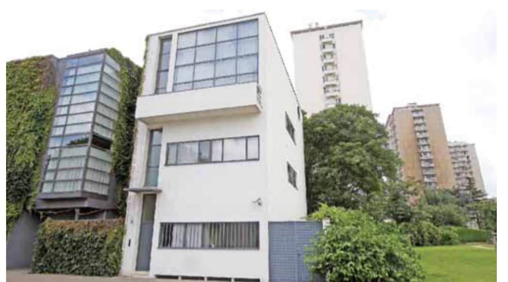
The Maison Guiette designed by Franco-Swiss architect Le Corbusier in 1926, in the district of Populierenlaan in Antwerp.
