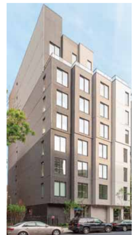
The micro apartment building Carmel Place in New York.
