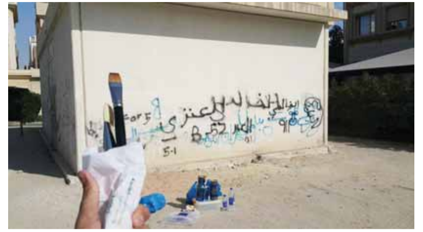
Power transformer (before).
