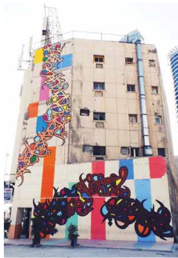
Graffiti covering the whole building.
