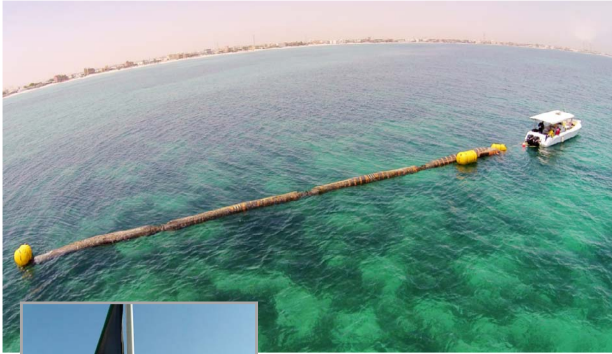
The Kuwait Dive Team removes an oil pipe in Khairan.
