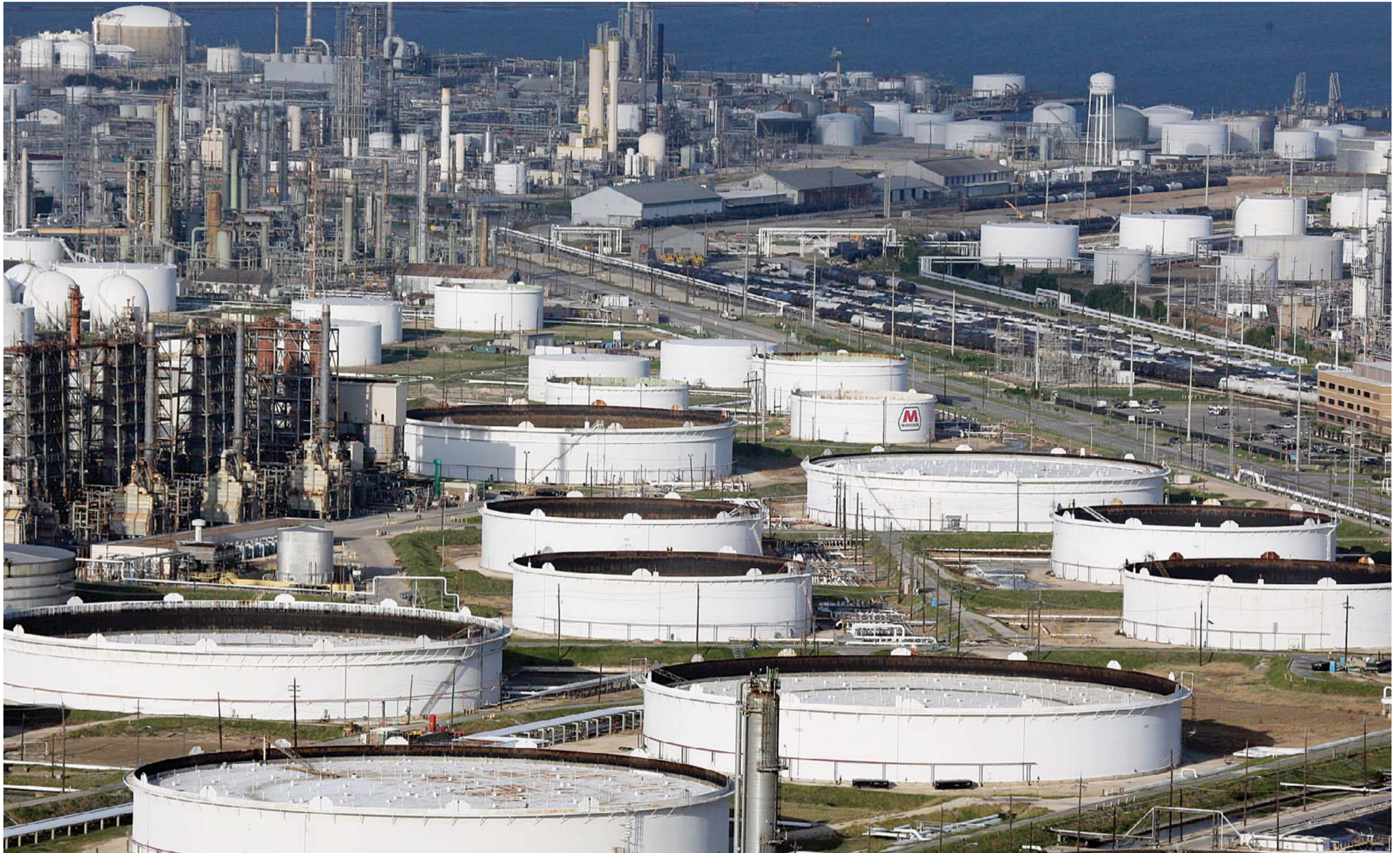
TEXAS CITY: Marathon Oil's refinery in Texas City, Texas. Seven of the 10 biggest losers in the S&P 500 in 2015 were energy companies. With crude prices at 11-year lows, the world's biggest oil and gas producers are facing their longest period of investment cuts in decades. —AP
