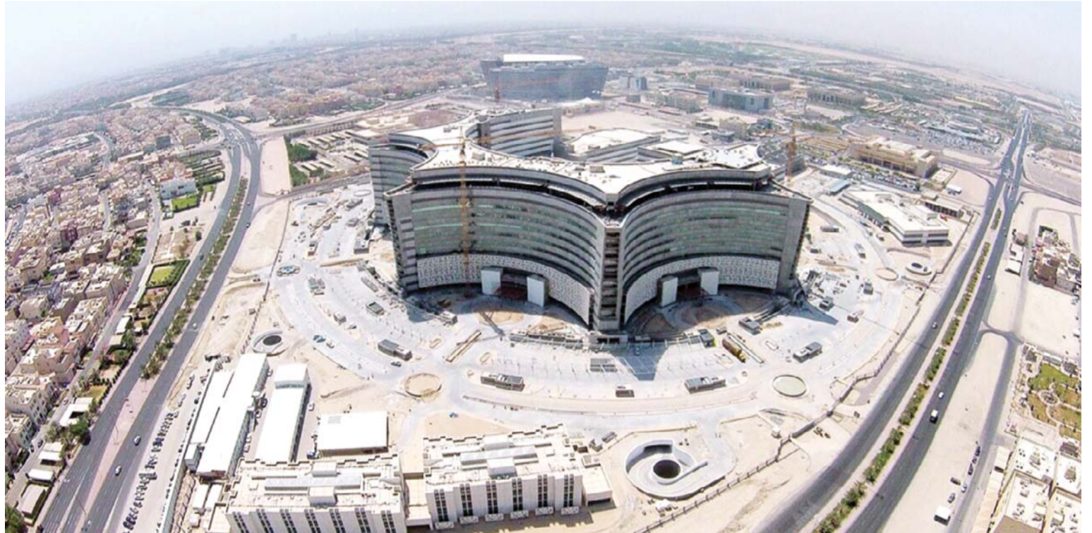
This file photo shows the Jaber Hospital under construction.
