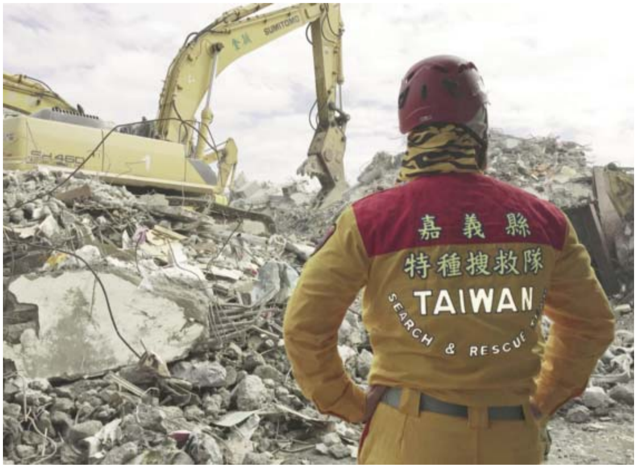
TAINAN: A member of rescue teams stands by as heavy excavation machinery continues to dig through the rubble of a collapsed building complex. — AFP
