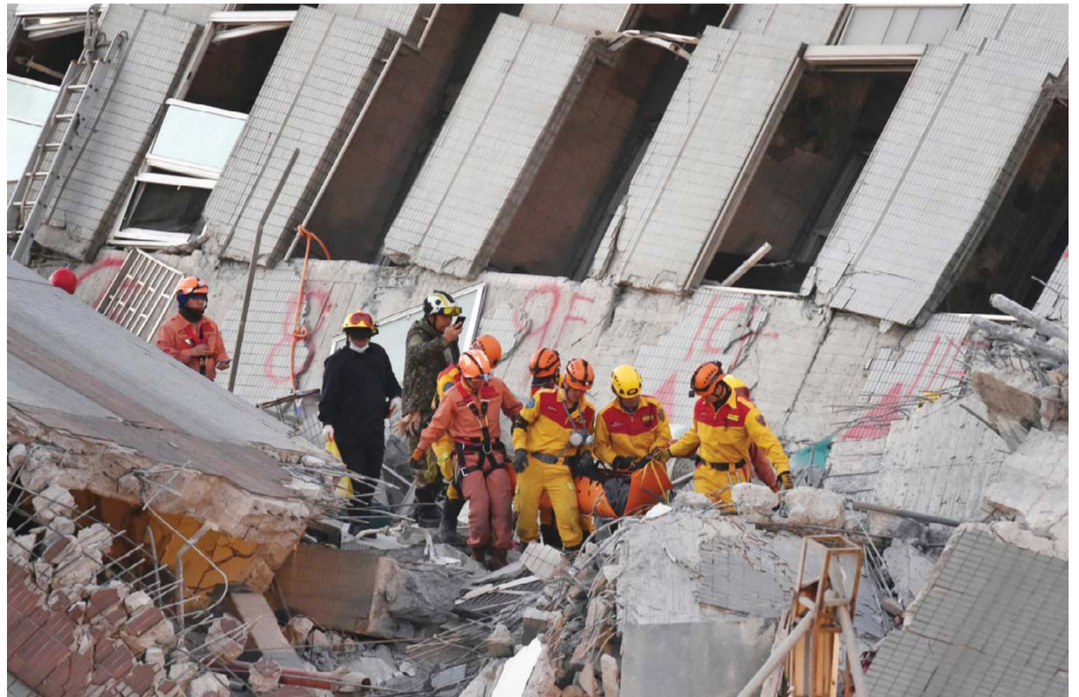
TAINAN: Rescue personnel bring down a Vietnamese national, identified as 28-year old Chen Mei-Jih, to safety after she was extracted from the rubble at the Wei-Kuan complex which collapsed in the 6.4 magnitude earthquake. — AFP
