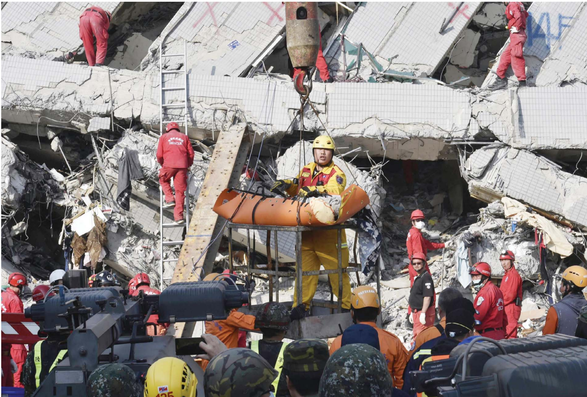
TAINAN: A rescue worker brings down a victim from the collapsed Wei Kuan complex building. —AFP
