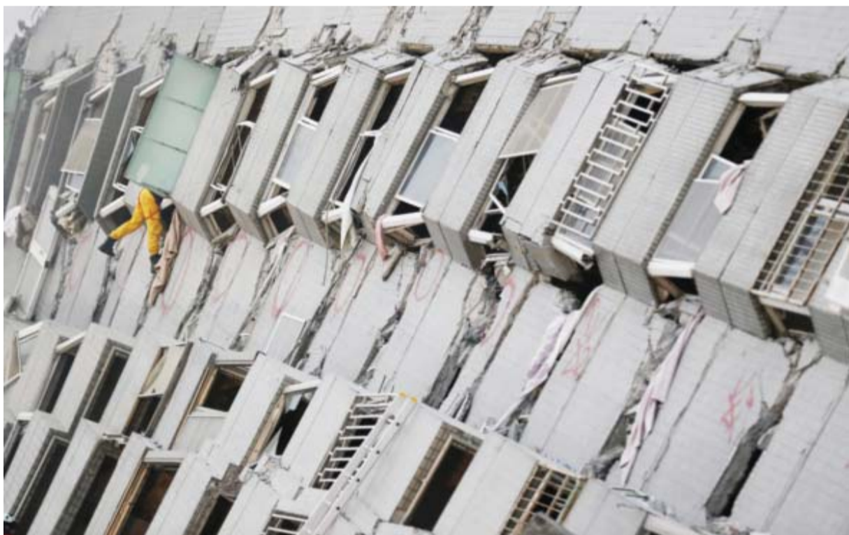
TAINAN, Taiwan: A rescue team member searches for missing people in a collapsed building after an early morning earthquake yesterday. — AP
