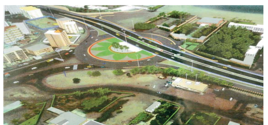
KUWAIT: This archive photo shows an artists' rendition of the planned renovation of the Bidaa Roundabout. — KUNA
